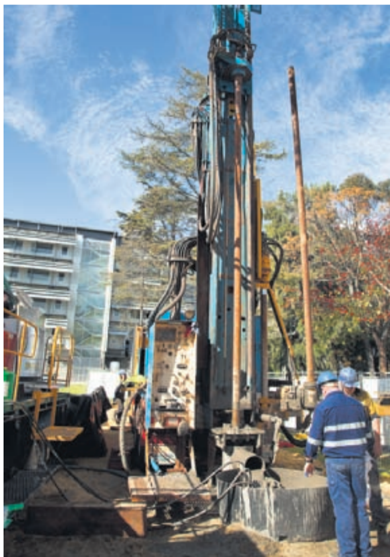
The exploration drill rig at UWA
